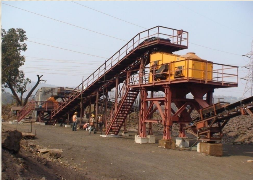
Stationary crushing & Screening Plant at TATA STEEL PLANT
